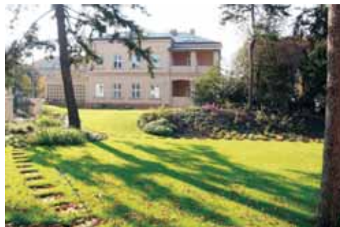
Rekonstrukce objektu Pelléova, 2004/ Reconstruction of Building in Pelleova, 2004
