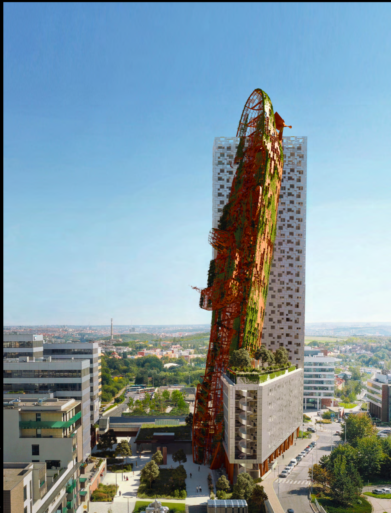
Top Tower, Praha 13, Prague 13
