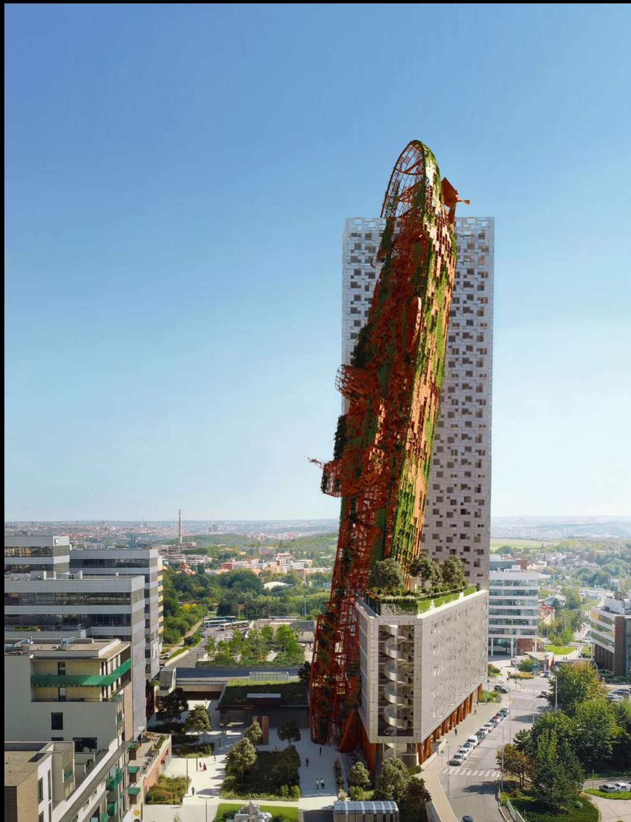
TOP TOWER, Praha 13, Prague 13
