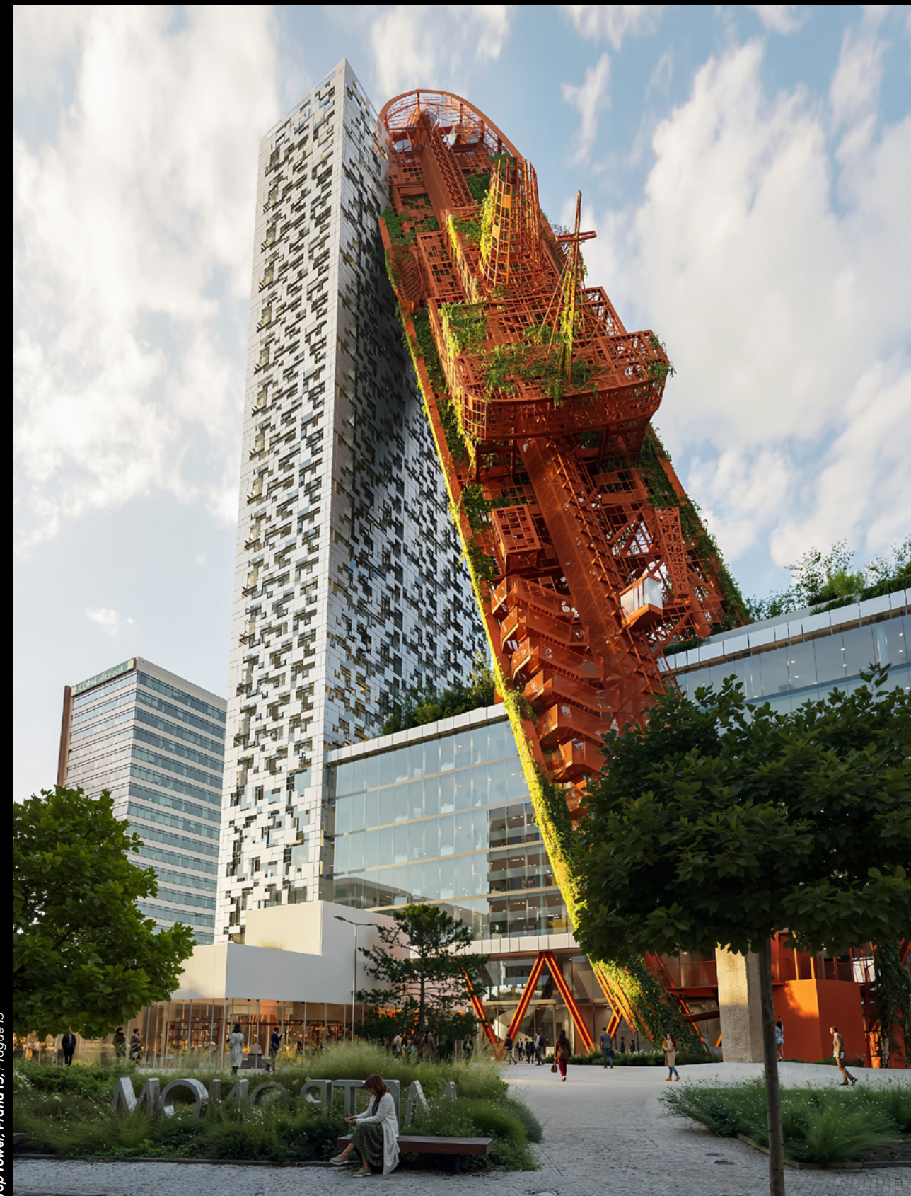
Top Tower, Praha 13, Prague 13
