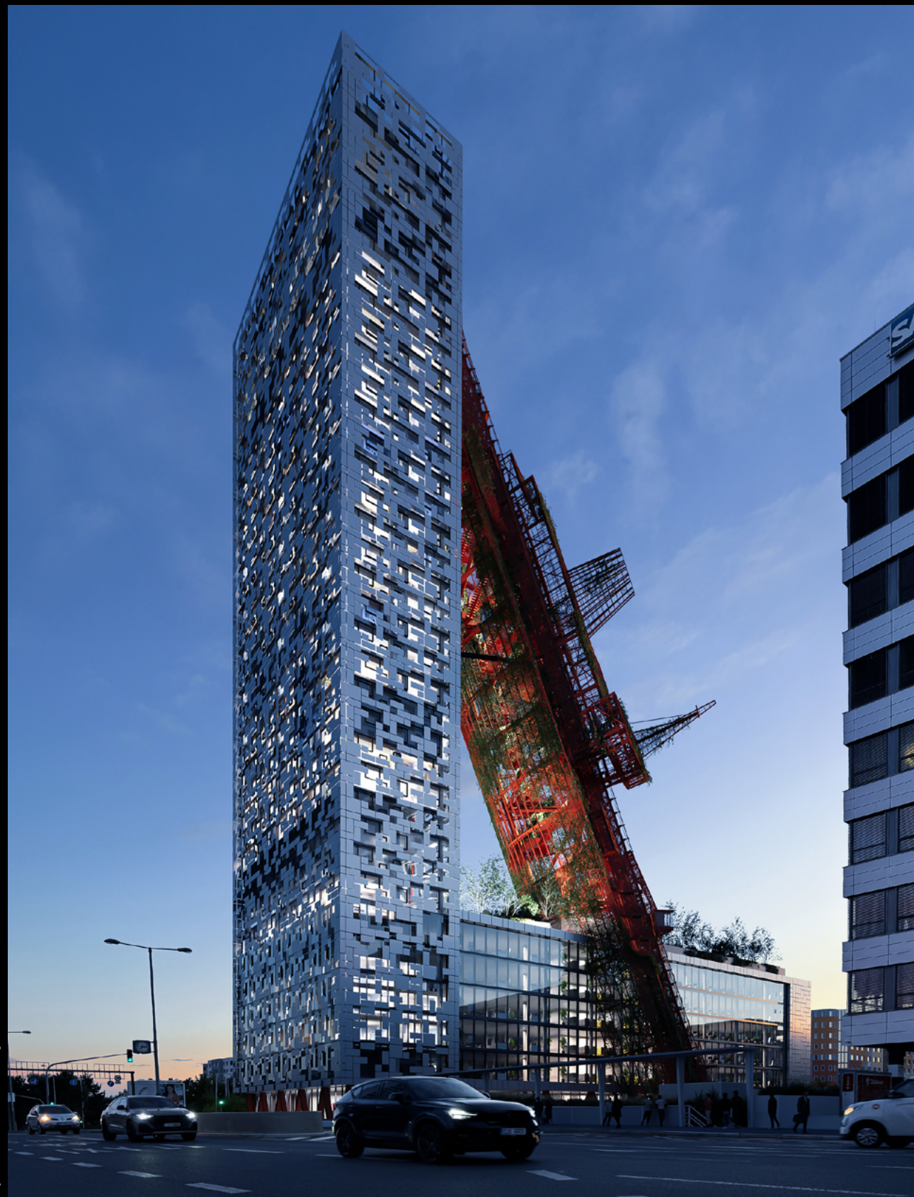
Top Tower, Praha 13, Prague 13
